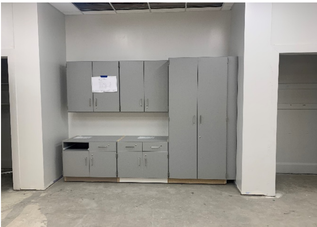
CES - Casework installation at classrooms
