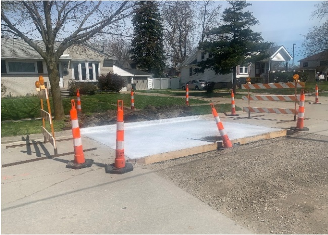
CES - Sitework along Phillips Avenue
