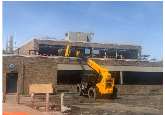
CES - Window Replacement at Cafeteria
